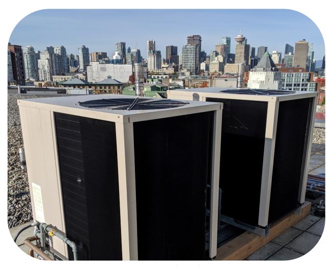
Image: GAHP units being commissioned at a facility for a FortisBC pilot project in Vancouver, British Columbia. Courtesy of Building Energy Solutions Ltd.
